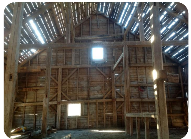
Second floor with metal roof removed
