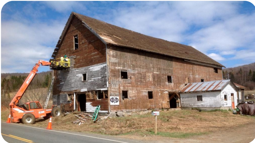
StoriedBoards reclamation of the gray clapboard siding
