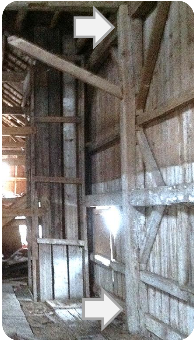
Left: slight gunstock post, with larger top than bottom Above: intricate beam braces
