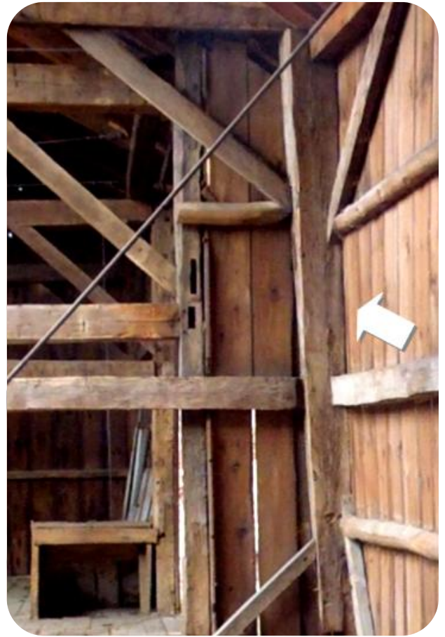
Gunstock Post, with its larger top than bottom
