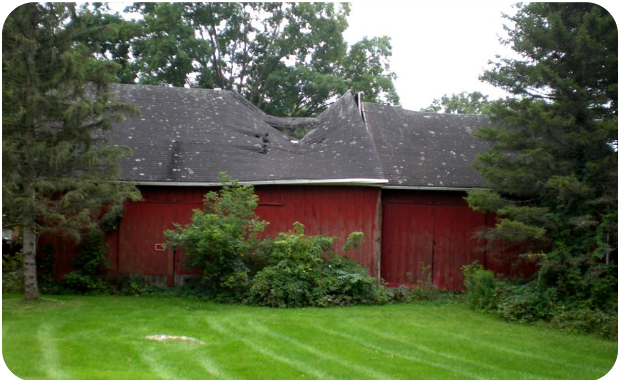
North side of the barn, showing failure of the roof
