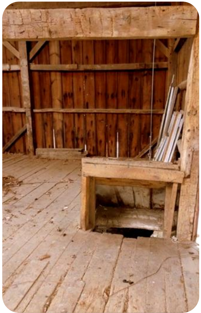
Thresher floor and hay chute
